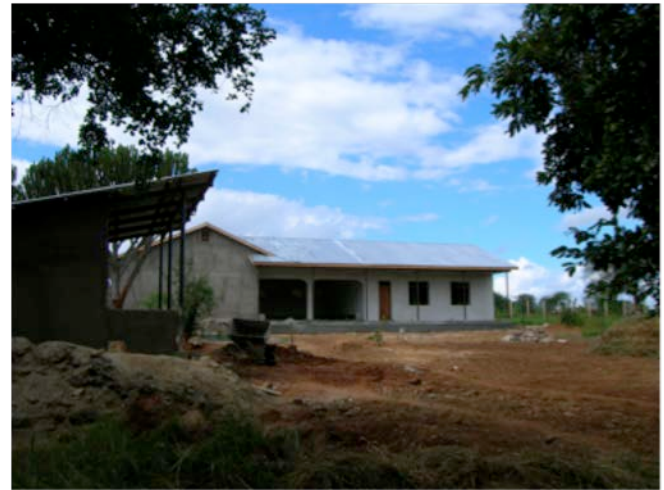
SONAB: the multi-purpose dining room, classroom and toilet block under construction
